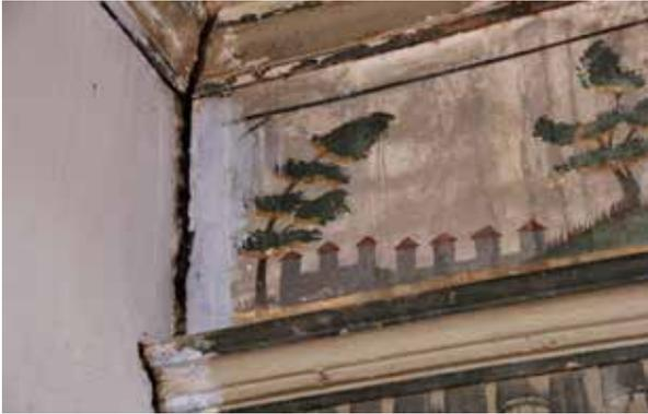
Fig. 16: Wall detachment and poor-quality paint layer
