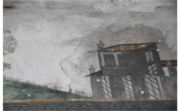
Fig. 17: Poor quality paint, cracks and soot layer
