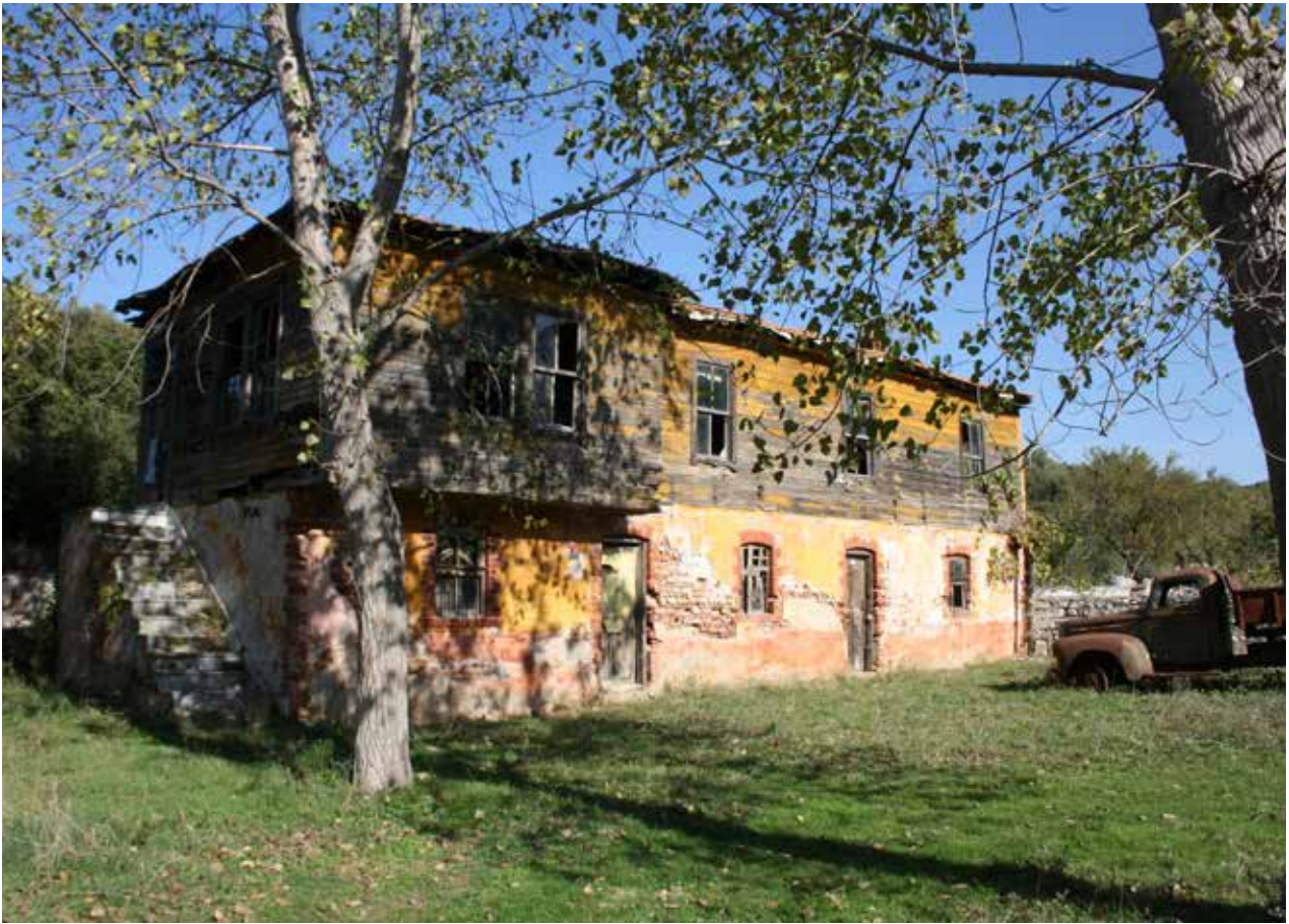
Fig. 2: Administrative building, southern and western façades
