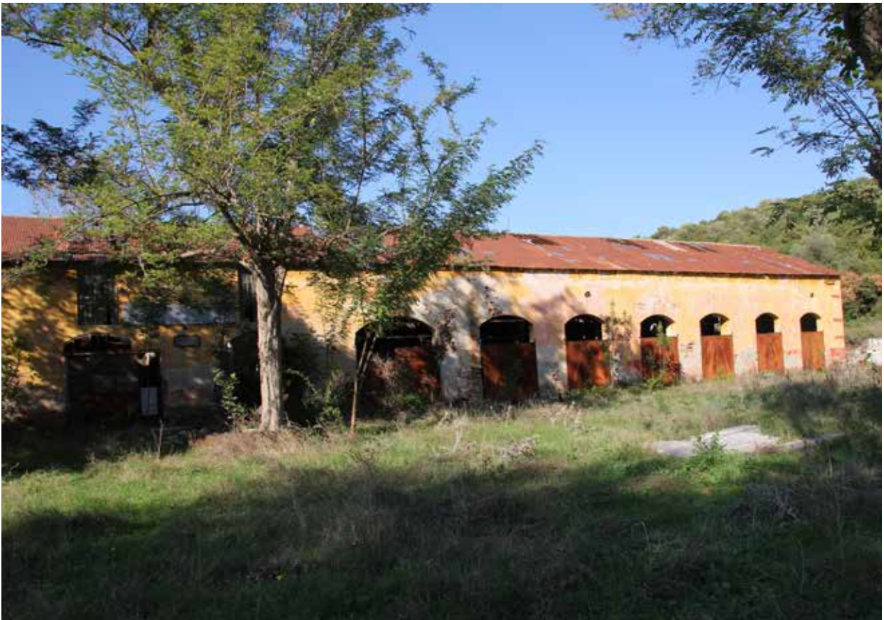
Fig. 3: Factory building, general view
