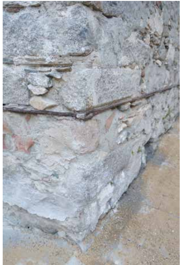
Fig. 3: Detail of masonry and iron bands
